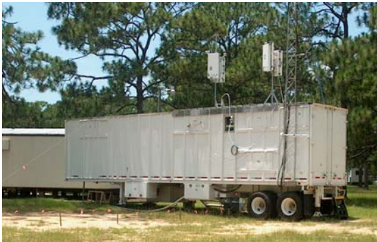
The MAQL fully deployed and operational at the OJ Semmes ES site on July 18, 2003
