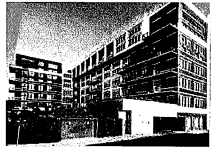
Parc Lofts Miami, FL 72 Loft Residential Units Project Cost: $9 Million Client: Urban One Development LLC
