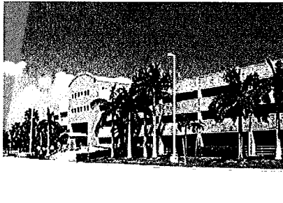
Port of Miami Parking Garage Miami, FL 2 Acres 720 Parking Spaces 4 Stories Project Cost: $4.5 Million Client: Miami-Dade County Seaport
