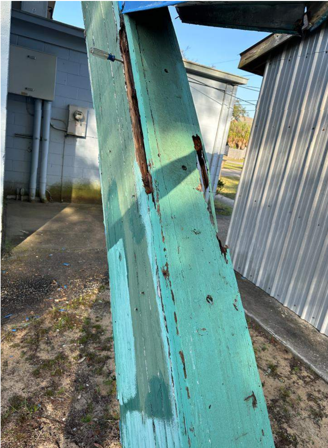
Arch #7; East End of Arch near NE corner of Bldg
