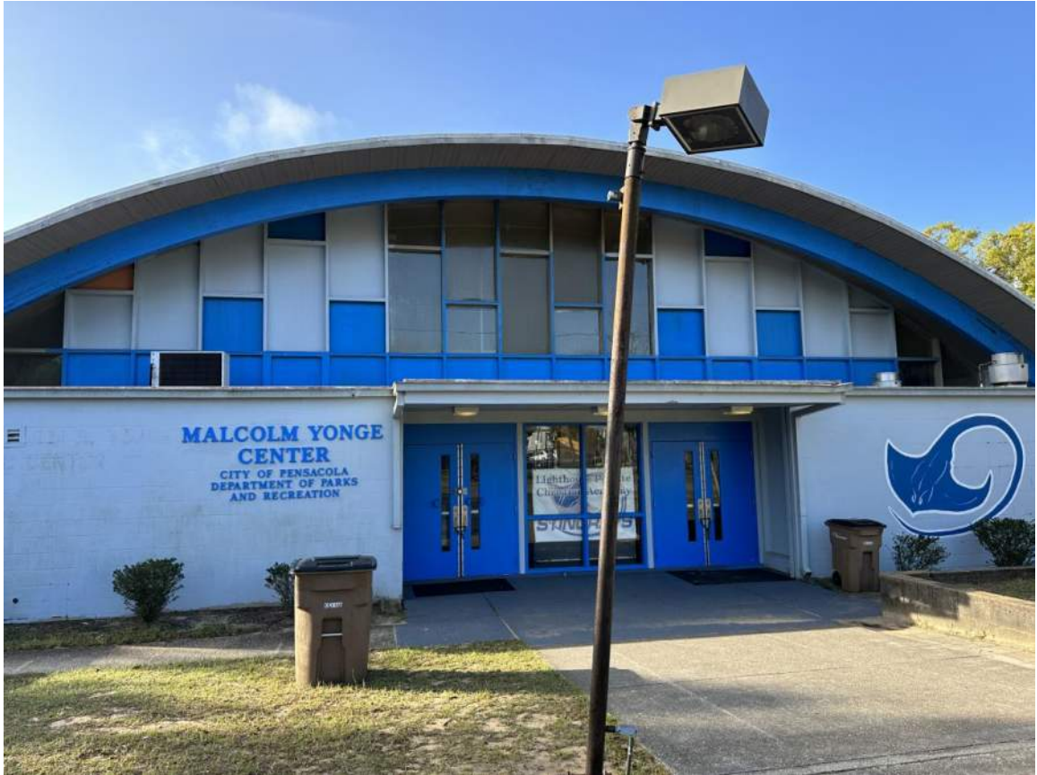
North Side of Building (Looking South)
