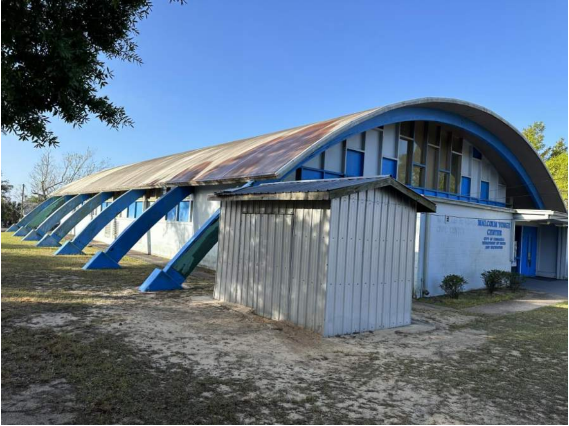
North Side of Building (Looking SW)
