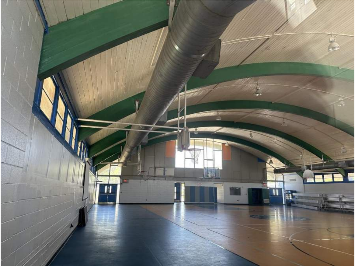
Inside of Bldg (Looking South towards south wall)
