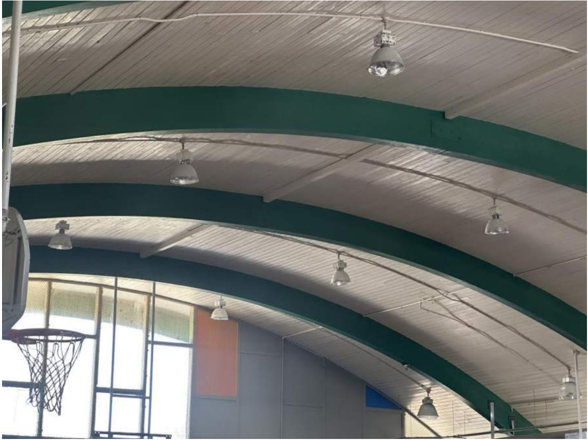
Inside of Bldg – Top of Arches (Looking South)
