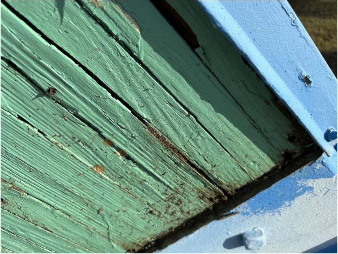
Arch #4 in Photo Foreground; East End of Arch
