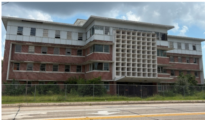
Vegetation surrounds a vacant structure on Palafox Street.
