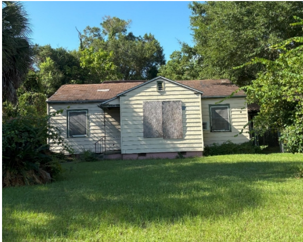
Left: Vegetation overtakes a single-family home. Right: A vacant home sits amidst robust vegetation.
