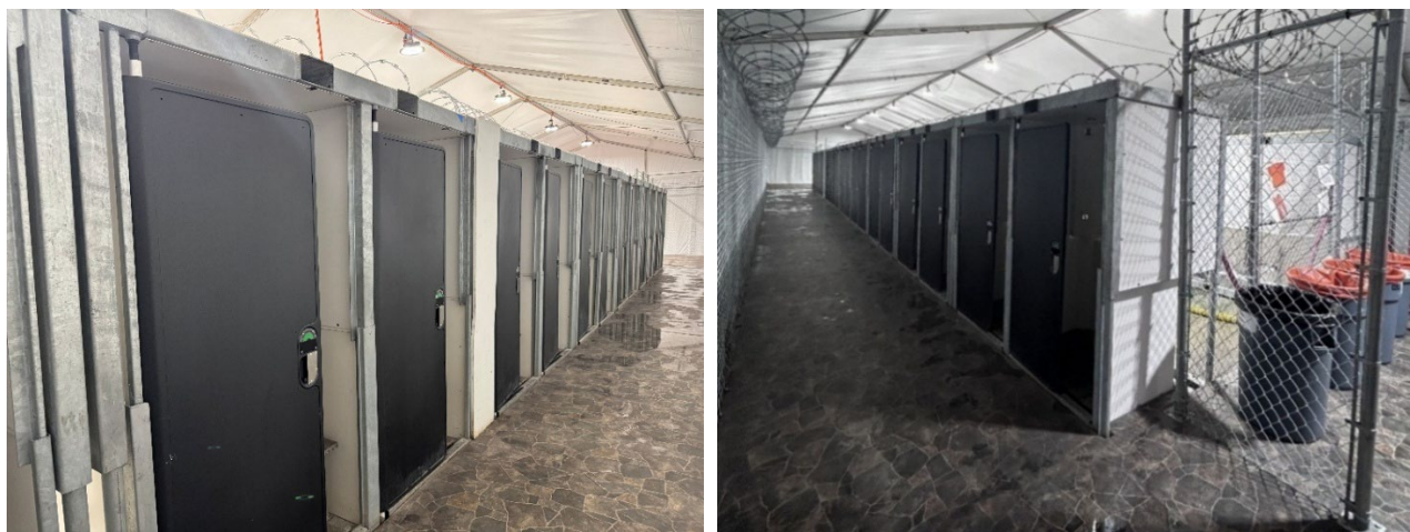
Figures 19 and 20. Shower Facilities; Observed January 21, 2026
